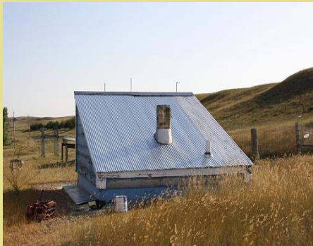
Bear Creek repair (what we can do about it)
