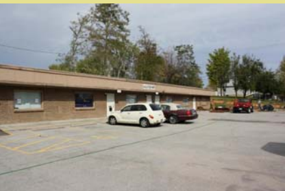
Another building and fence being installed
