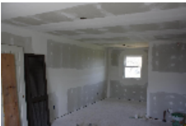
New drywall & window
