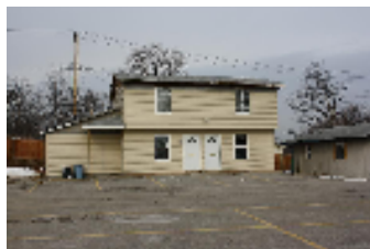
Exterior after — almost complete
