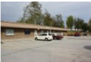
New doors, roof and interior.
