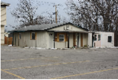
Windows and doors in, ready for siding.
