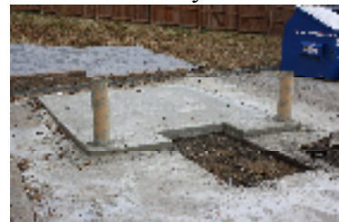
Oasis - concrete for freezer
