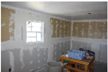
Oasis - wall repairs
