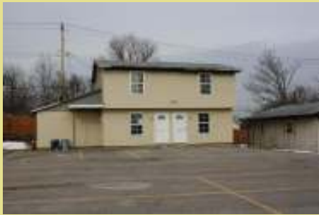
Oasis building being restored.
