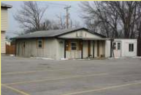
Another Oasis building ready for siding.
