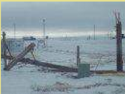
No electric knocked out water system
