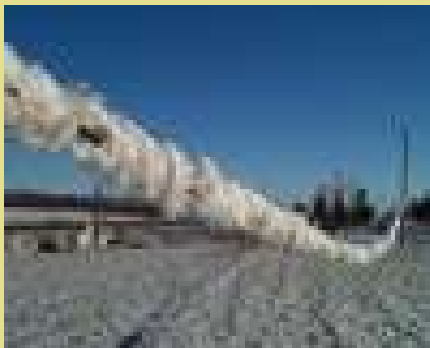
Reservation: downed power lines.
